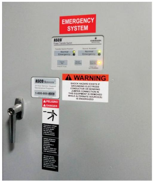
Photo 3. This transfer switch shows examples of how both labels are implemented in an end-user application.
