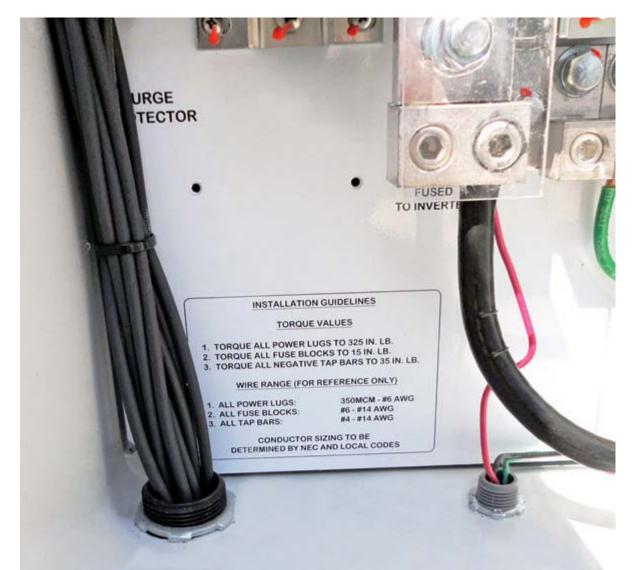
Photo 2. Many manufacturers will place a "torque" label next to or adjacent to the equipment to make it easier for the inspector — or those doing service — to maintain the integrity of the system.
